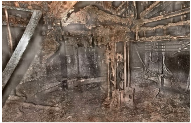
Fig. 4. Inside the pressure containment vessel of the Unit 2 at the Fukushima Daiichi: melted fuels (brown elements are believed to be fuel debris) have fallen from the pressure vessel. Source: International Research Institute for Nuclear Decommissioning (IRID).
