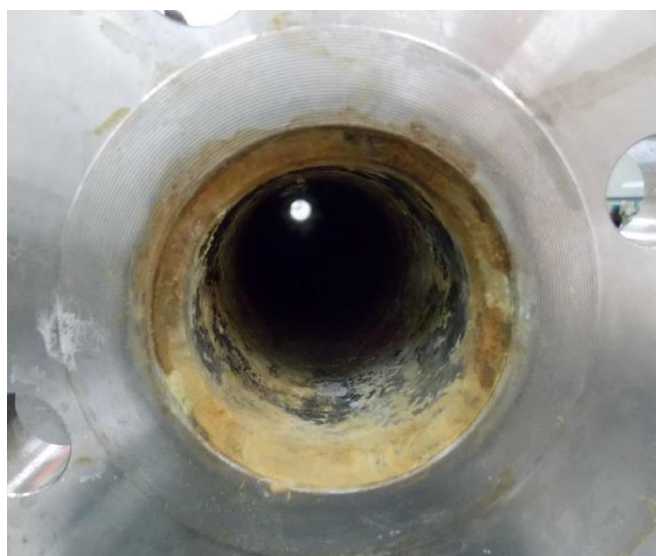
Figure 15 - corrosion within the inlet of the test rig column during acute HF testing Intersorb
