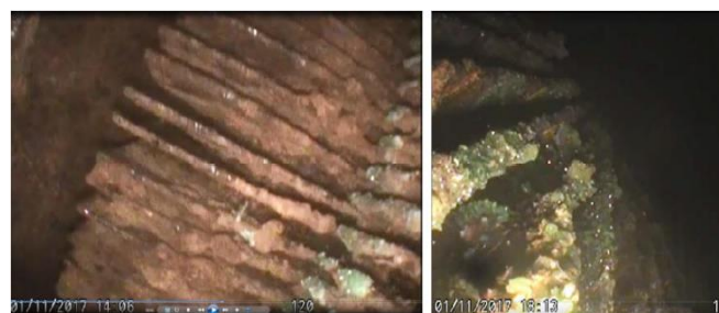
Figure 1 – Internal inspection pictures of cooler / condensers' heat exchanger surfaces
