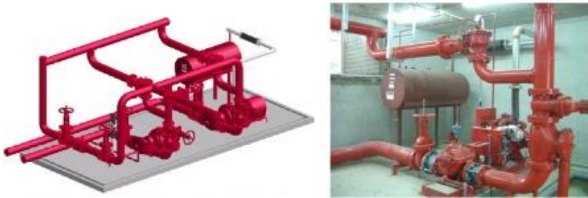
Figure 8 - Fire suppression system decomposition, motor, foam tank and Generator (Tserng et al., 2011)
