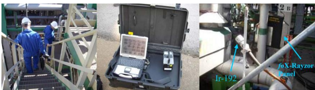
Figure 39 Setups of the portable digital radiography system in TOTAL refinery [188]
